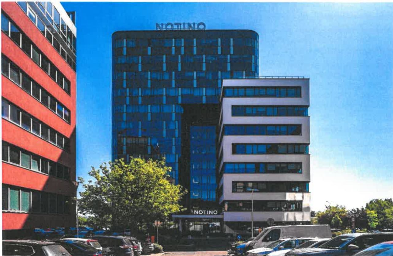
Budova E – BBP OFFICES
