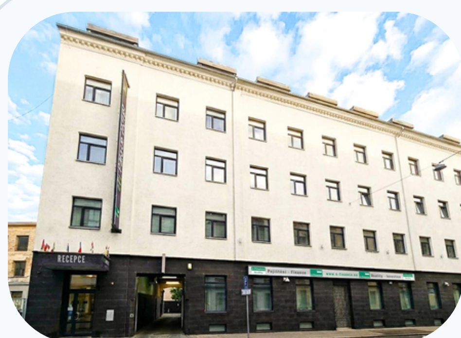
EFI Palace, Brno
